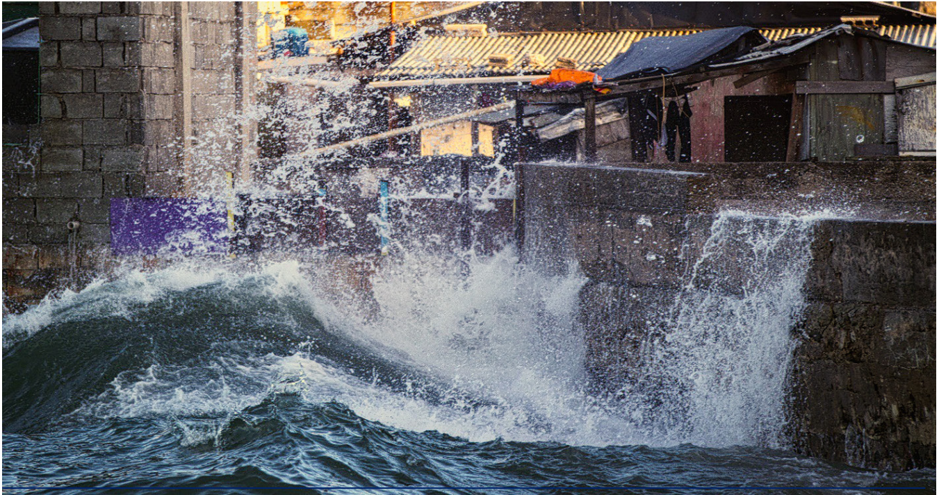
Waves splashing over a seawall near a home in Majuro during a king tide event in September 2019. Image credit: David Krzesni.
